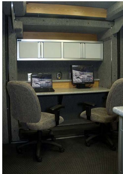
Two-man communications console is positioned in the slide-out room opening the interior up for traffic. Note solid-surface desk and aluminum cabinets with integration wiring access panels
